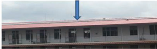
100 meters of Solar Panels 75 X 300W ; 45 X 255W
