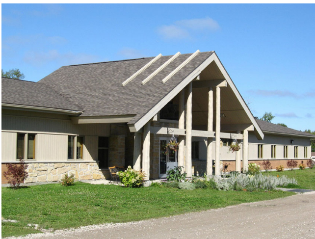
Figure 1 The Share Office Building.
