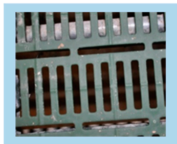
Figure 2. Plastic slatted floor with 10 mm slat width, 10 mm slot width, and 50% perforation—B (commercial plastic slatted floor for pigs, MIK, Siershahn, Germany).
