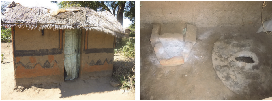
FIGURE 1: Fossa antenna superstructure and inside the latrine in Chikwawa.
