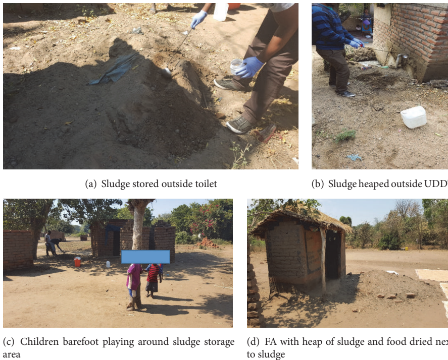
FIGURE 4: Faecal sludge storage and possible exposure pathways.
