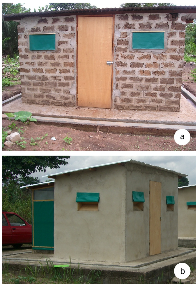
Figure 1 Experimental huts used in the study located in the M'Bé site, near Bouaké in central Côte d'Ivoire. The experimental huts comprised a sleeping room and a veranda. The walls of the room were either made of concrete bricks coated with cement (a) or wood structures coated in dry mud – locally called banco (b).
