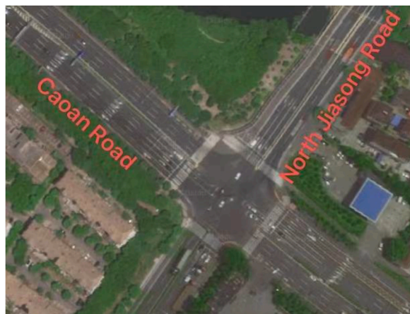
Fig. 3. Cao'an road – Jiasong north road intersection.
