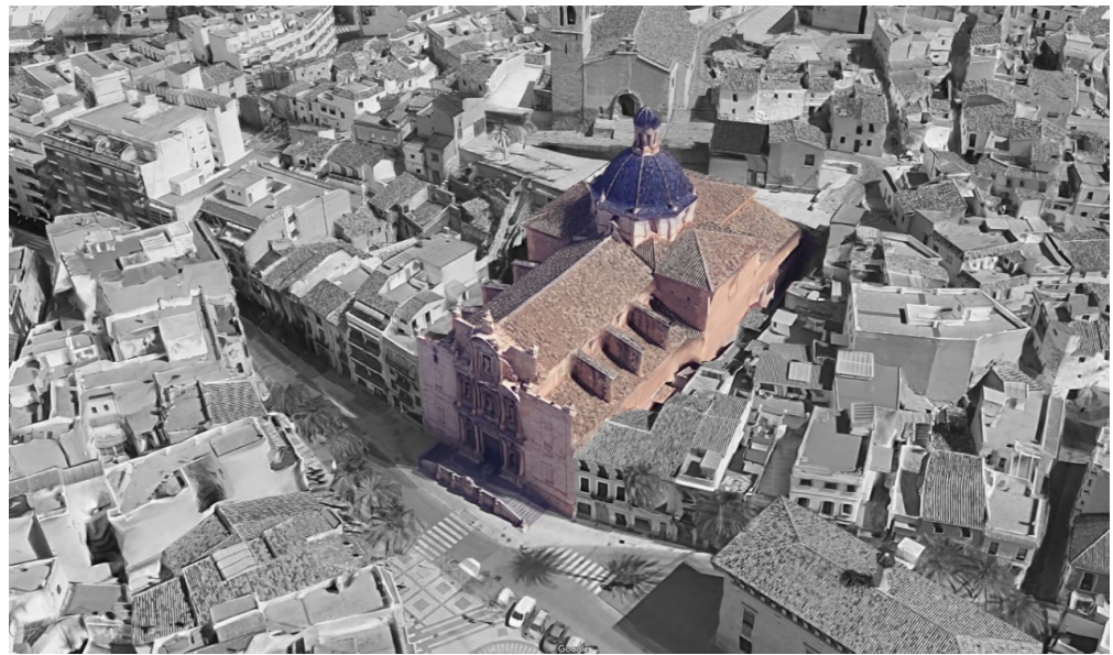
Figure 1. Aerial view of the building (Source: Google & National Geographic Institute of Spain).
