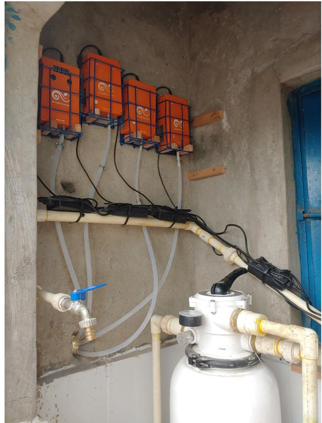
**Figure 4. Ozone generators in the utility housing.**
