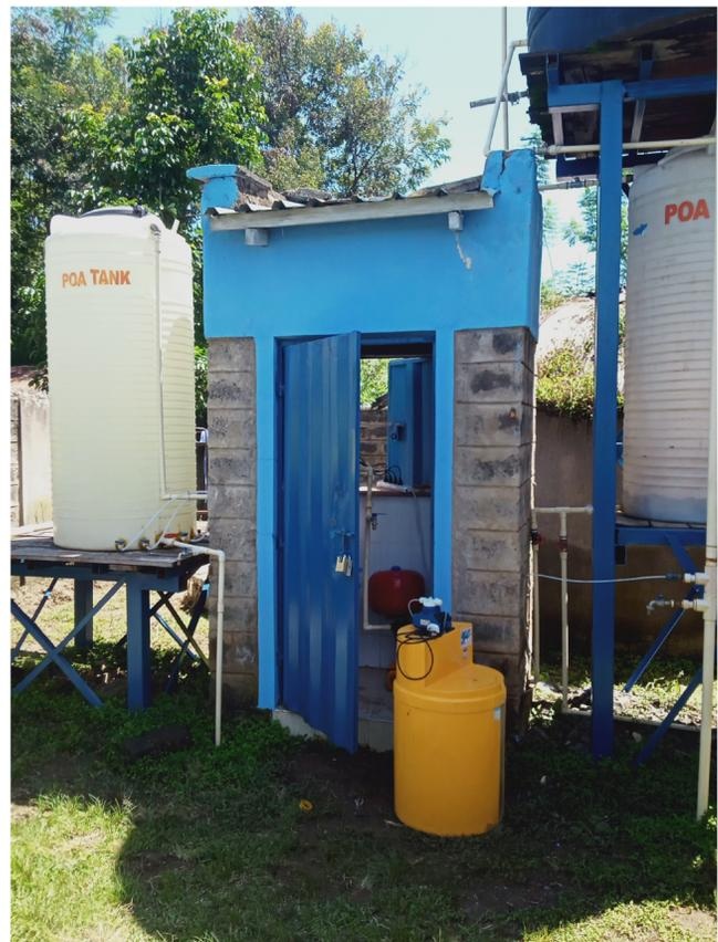
**Figure 2. Utility housing.** Upper right: The large black tank on the right is the settling tank; Right: The white tank is the balance tank; Left: The white tank is the ozonation tank. Tubing carrying ozone to the diffusers (not visible) can be seen entering the tank. Yellow container in the foreground contains alum.
