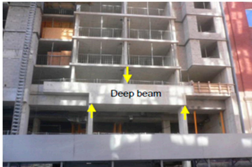
Figure 1. Deep Beam in a multi-story building [2].
