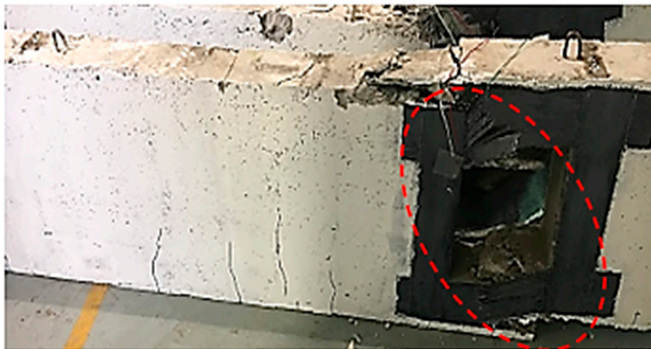
Figure 14. Failure mode and cracking pattern of deep beam B3c.
