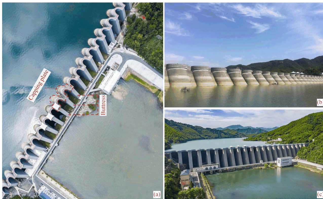
Figure 1. Foziling multi-arch dam: (a) top view; (b) upstream view; (c) downstream view.
