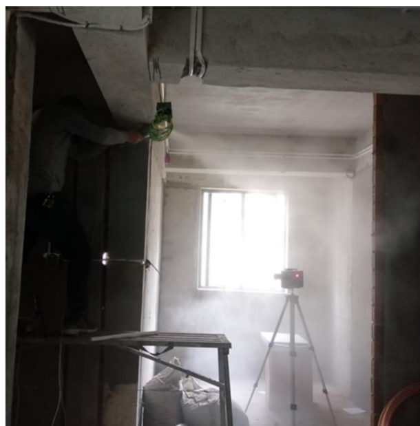
Figure 1. Dust detection carried out in the interior construction site.
