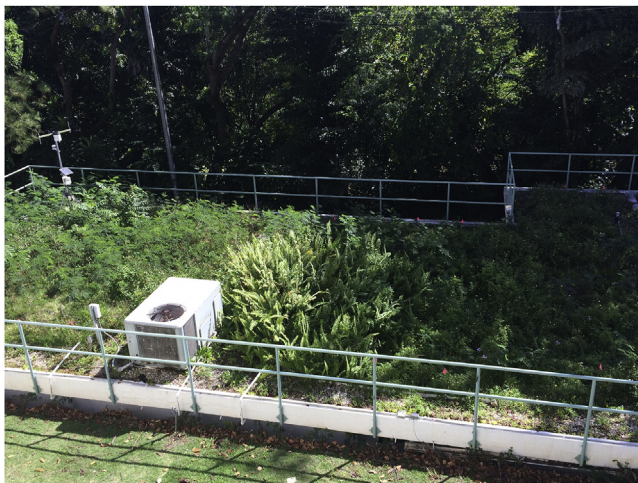
Figure 2. GIS Laboratory (Green Roof # 0–3) years after installment with no maintenance (Image by Author).
