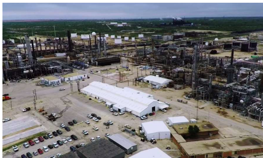
Figure 8. Oil Refinery in Howard County, Texas (image from Google).
