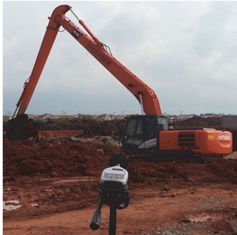
Fig 7. Mapping Area of Drainage Excavation.
