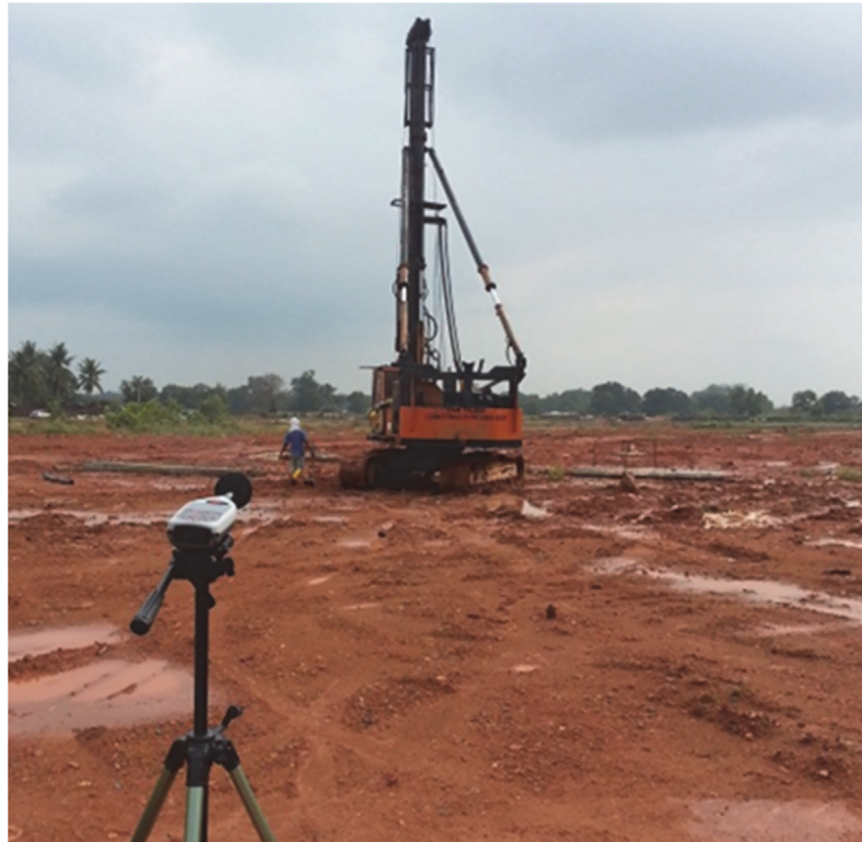
Fig 6. Mapping Area of Piling Activity.
