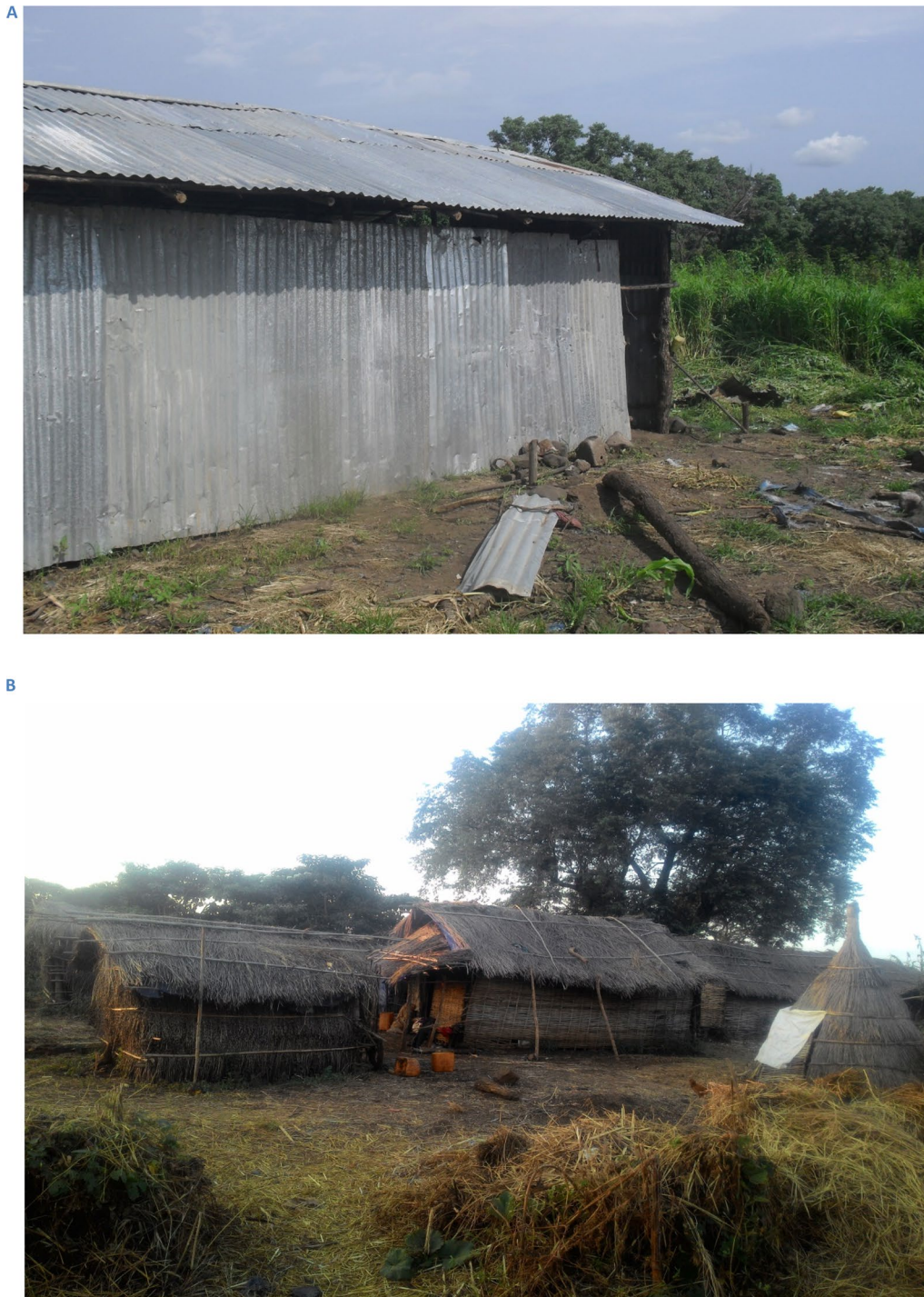
Fig. 2 Seasonal migrant workers stay in temporary shelters on agricultural farms. Typical shelters are made from a variety of materials including iron sheeting (A) and grass (B)
