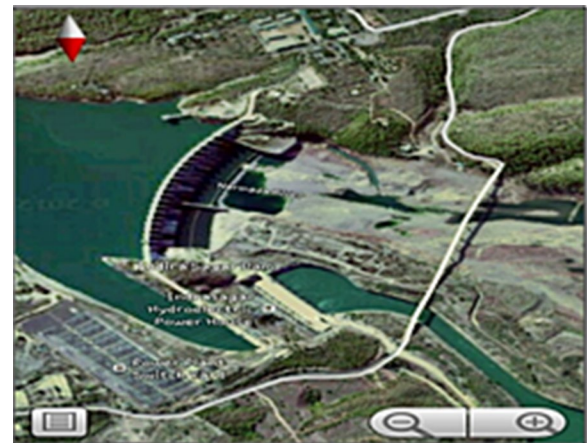
Fig. 1 ISP Dam site, Narmada Nagar, MP
