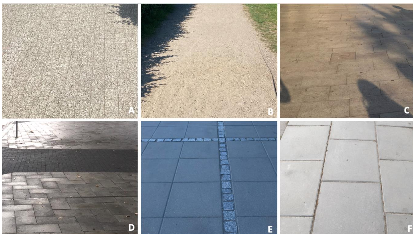
Figure 3. Various combinations of pavement surface subjected to perception analysis in the survey (A)—small-sized concrete paver, (B)—mineral surface, (C)—stone pavement, (D)—medium-format concrete paver, (E)—large-format concrete slab combined with granite paving pattern, F—large-format concrete slab. (source: processed by the authors).
