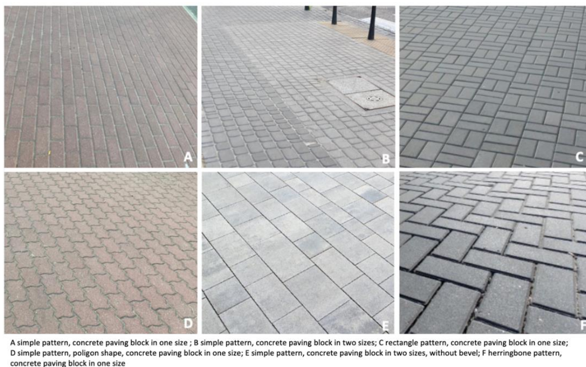
Figure 12. Concrete paving block patterns (A–F) analysed in correspondence with the analysis in Figure 11 (source: processed by the authors).
