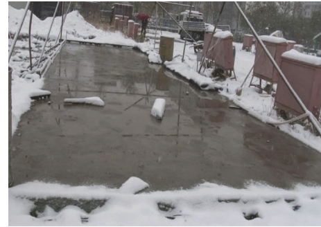
FIGURE 10: Snow melting performance of heat pipe pavement on 22 November 2015.
