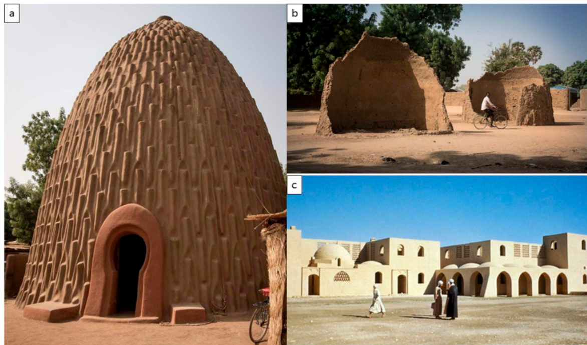
Figure 2. Vernacular clay architecture in Africa with simple building technologies: (a) shows Mousgoum houses built with clay by manual methods, while (b) exhibits the ruins of some of these Mousgoum houses due to cracking or poor rain resistance due to the hydrophilic nature of clay materials, and (c) exhibits earthen architecture by Hassan Fathy in New Gourna village in South Egypt, exploiting the passive cooling nature of clay materials through employing it in the design and construction of passive cooling Islamic architectural elements [29] (Photos: Institute of Nomadic Architecture. http://artsection.org/mousgoum.html ).
