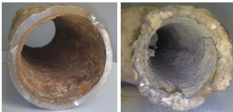
Figure 1 The corrosion in the re-injection pipes of the oil field.
