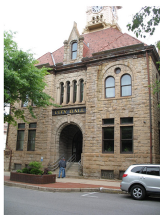
High water marks from the three biggest floods that have struck Johnstown (City Hall photos by N. Coleman).
