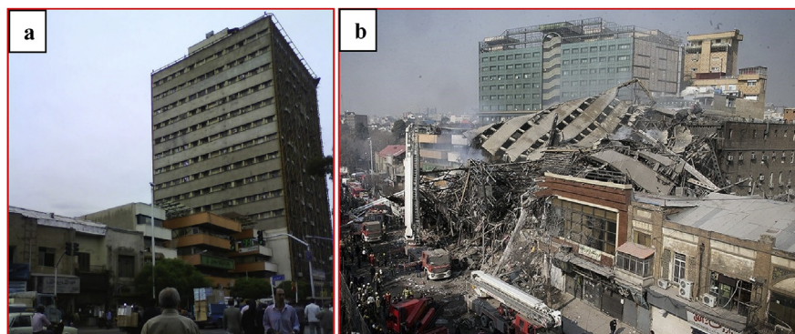
Fig. 1. The Plasco building in Tehran (a) before progressive collapse [5] (b) after progressive collapse [6].
