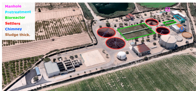
Figure 7. Aerial view of the WWTP used as test site, with the main odor sources highlighted in different colors
