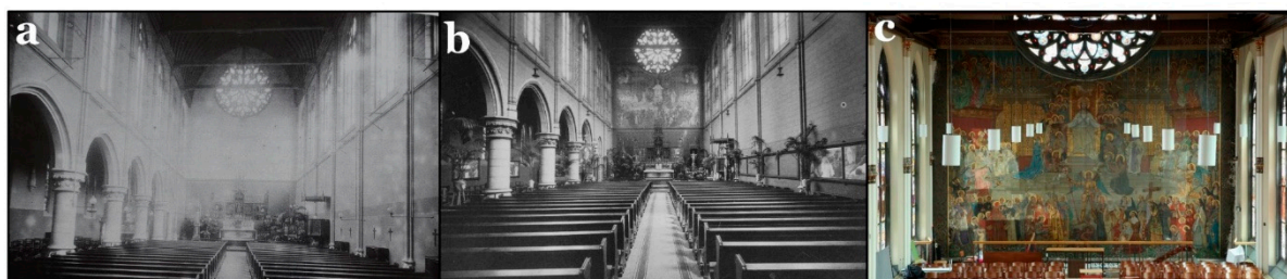
Figure 1. (a) A black and white photograph of the chapel in 1897 in the Sint-Jan Berchmanscollege, when the wall painting was not yet executed. (b) The chapel in the 1930s, after Ernst Wante created the wall painting. The chapel was not yet divided into two floors at that time [33]. (c) A photograph of the wall painting in 2017 showing its state before conservation. The wall painting is now found on the top floor of the chapel.
