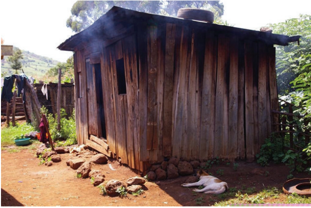
FIGURE 1: A typical rural Kenyan cookhouse with a small window for ventilation.
