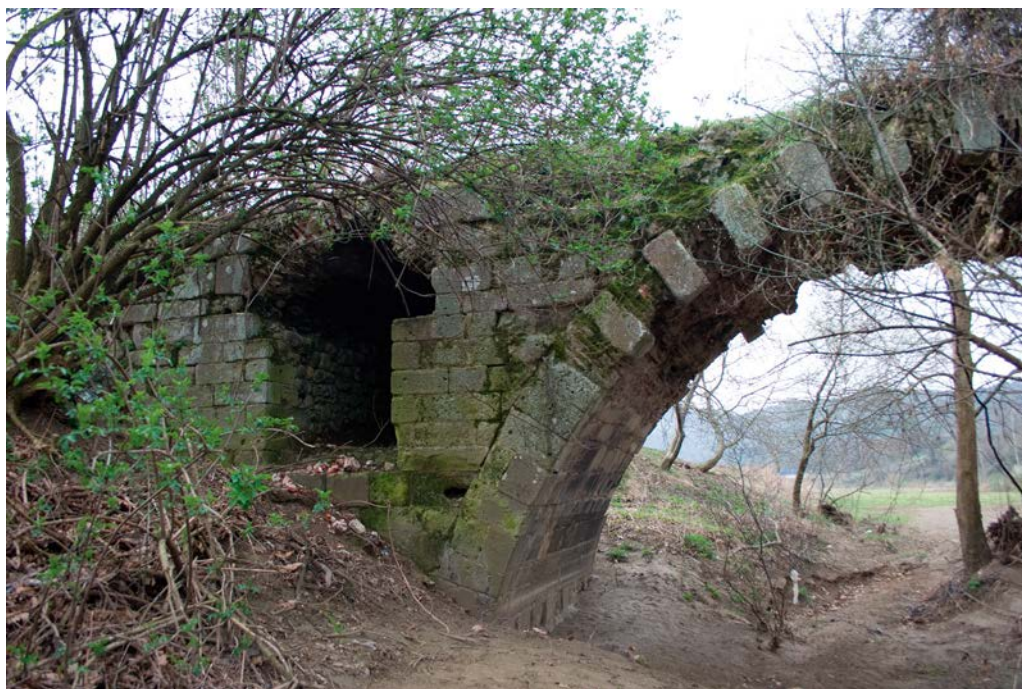
Figure 5 The Aesepus Bridge near Gönen, Turkey, westernmost arch of the eastern abutment and vaulted chamber, view from the north (photographer: Galina Fingarova).
