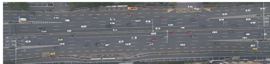
Figure 3. Aerial view of the urban expressway at a weaving section.
