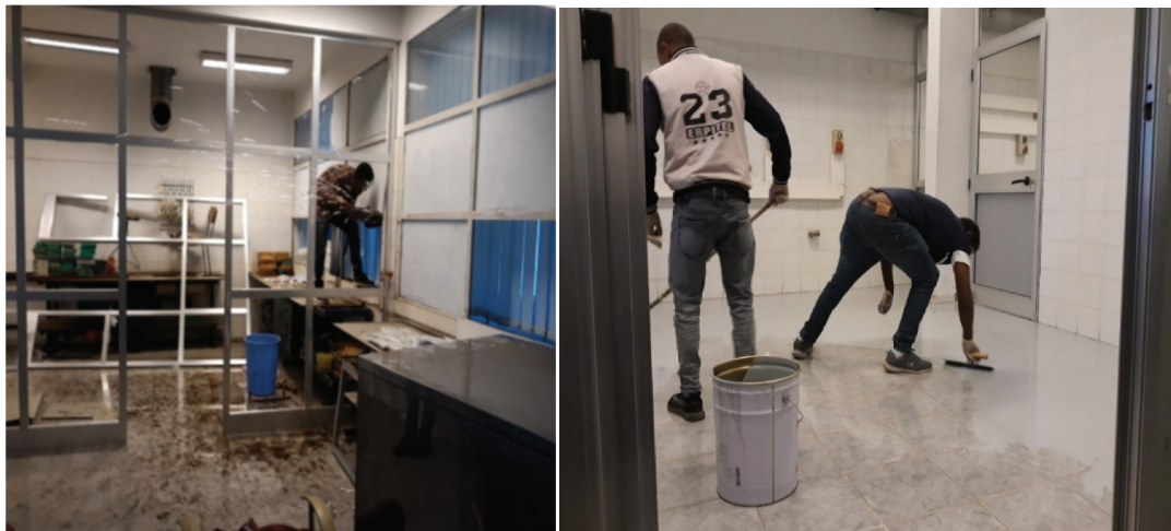
a) Room preparation for aluminium partition b) Epoxying the room
