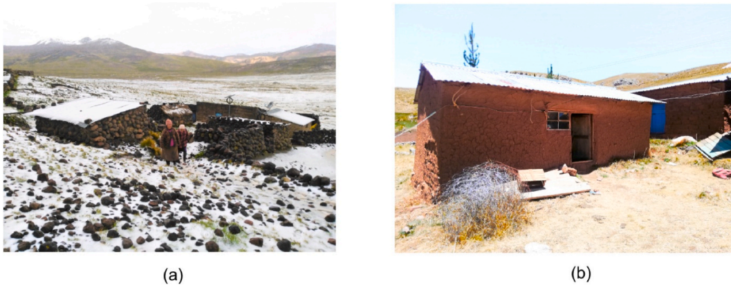
Fig. 1. (a) Household settlement formed by multiple huts and (b) typical mud-brick hut in the rural Peruvian mountains.
