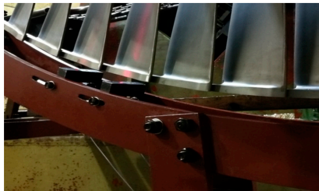
Figure 7. Installations of fiber optical sensors.
