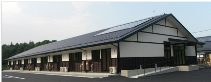
FIGURE 1 Front view of Idobata Nagaya . The building style is known as nagaya , a rowhouse commonly inhabited by ordinary people in downtown areas during the Edo period. Five buildings containing 58 units were built in Soma City after the earthquake
