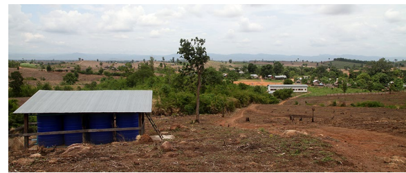
Fig. 1 Three water storage tanks were installed by the study team covered by a corrugate iron roof, which are a part of the improved water supply system provided as a community incentive to the village in the background
