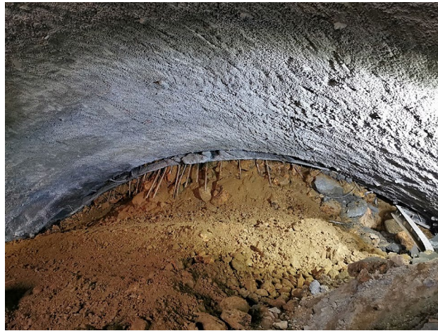
Figure 7. Tunnel collapse.
