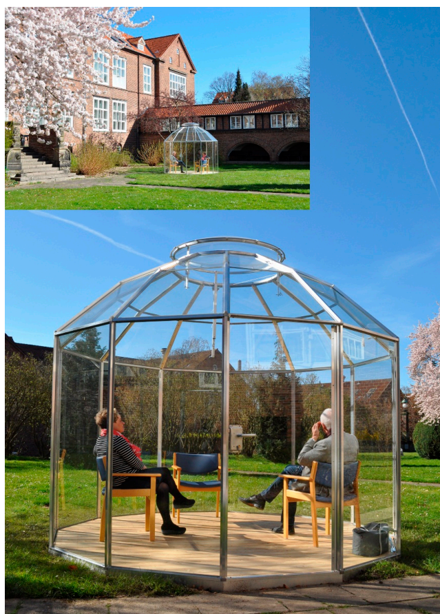
Figure 5. The greenhouse is constructed of one layer window glass with acrylic at the very top.
