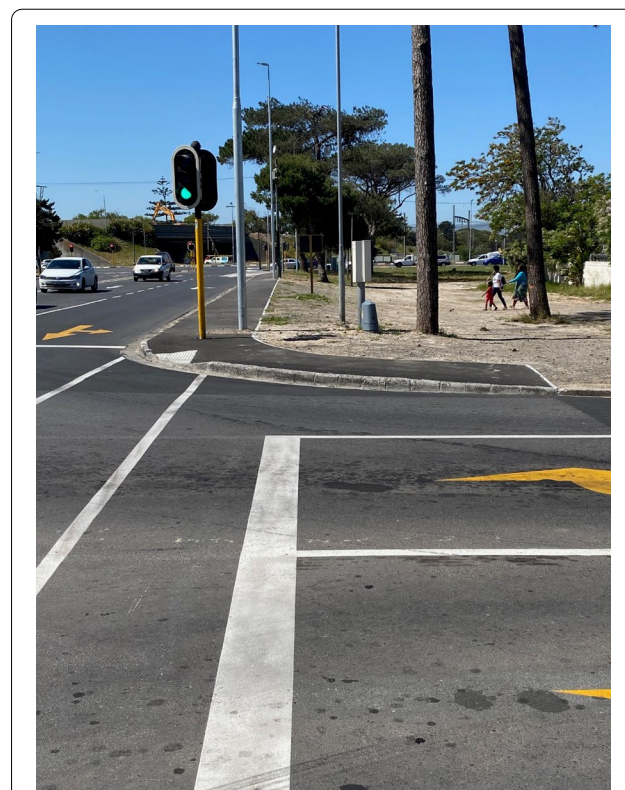
Fig. 6 Picture of an intersection in Cape Town, refurbished in 2020. Source: Picture taken by author
