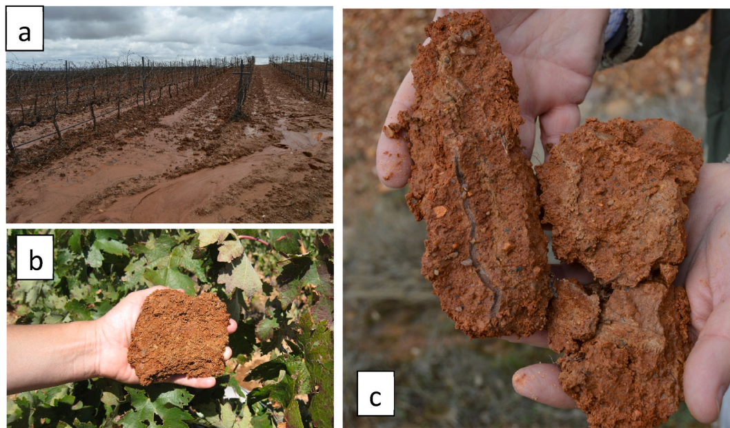
Fig. 4. a. Temporary hydromorphy and poor permeability; b. Ferruginous pseudo-crusts formed by iron oxides that act as cement; c. Signs of a pseudogleyization process in root channels.
