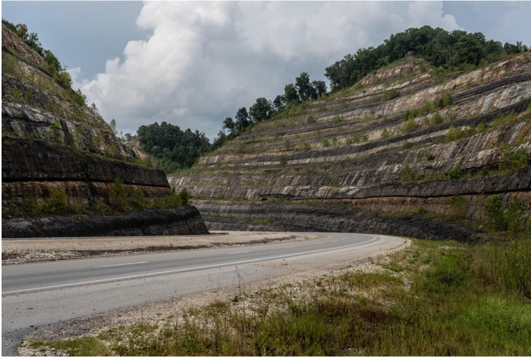
Figure 2: In eastern Kentucky, even basic infrastructure requires colossal feats of engineering. Modernization projects alter the landscape in unmistakable ways, leaving visual evidence of the tension between preservation and progress. Photo credit: Melanie McComsey.
