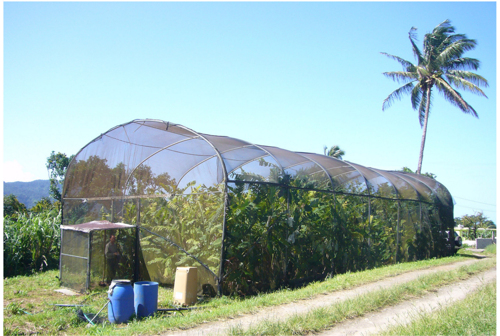
Fig 2. Enclosed Heliconia garden on Dominica. The dimensions of the screenhouse are 30 m x 10 m x 7 m.
