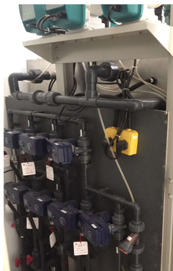
Figure 3. Pipeline distribution control system.
