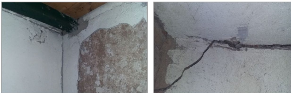
Figure 3. Inspection of grooves, holes, and cracks in walls.
