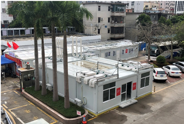
Fig. 3. Top view of the prefabricated negative pressure isolation medical unit.
