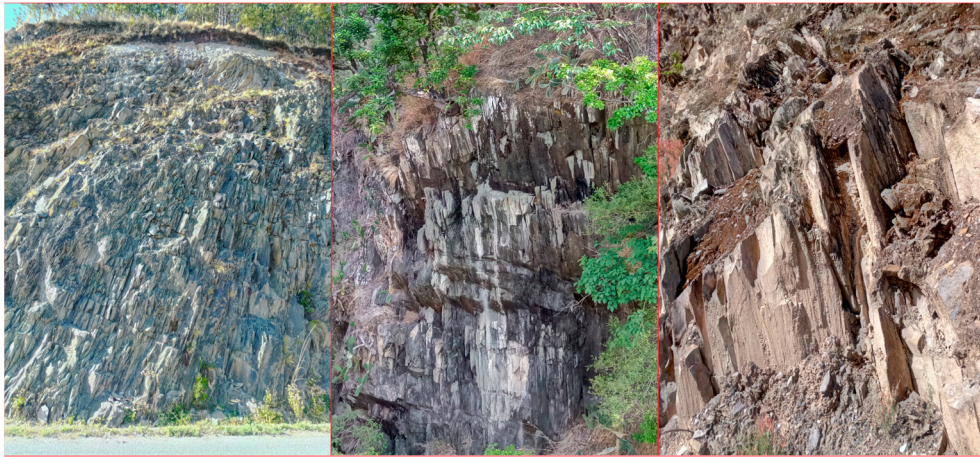
Figure 2. Exposed rocks of reservoir bank slopes in Miaowei reservoir area.
