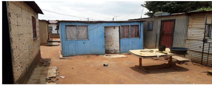
Figure 5. A typical backyard shack in the Kathorus area, shacks are usually no older than 10 years. Each backyard shack houses between one to three occupants. Shacks are usually made with corrugated iron and any scavenged materials. The number of windows was not standard, they were between 2 and 3. Shacks generally had a floor area of about 20–25 m 2 .
