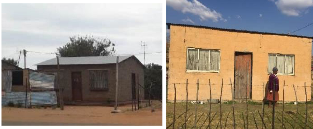
Figure 6. Examples of typical RDP houses in Wakkerstroom; the houses were constructed in late 90's to early 2000s with maxi brick and corrugated iron roofs (left), and the house at the right is an example of earlier (1994) RDP constructions with asbestos roofing and only one door at the front of the home. The houses had similar dimensions to those found in Kathorus.
