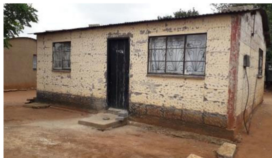
Figure 7. Apartheid era (matchbox) houses found in eSizameleni (Wakkerstroom), with a surface area of 40 m 2 . The houses had either asbestos or corrugated iron roofing with 2 doors and 3–4 windows.
