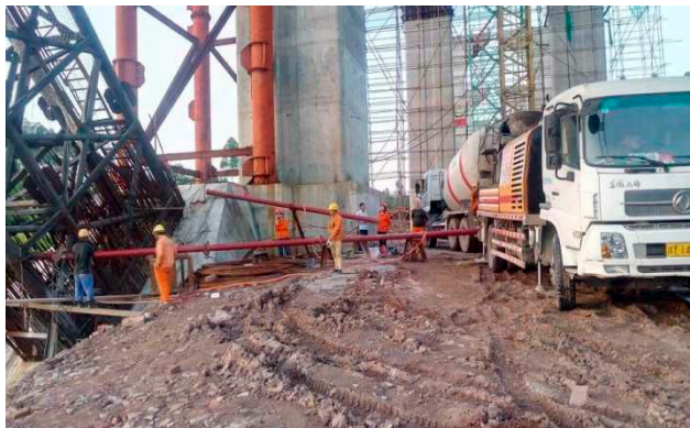
(b) Concrete pouring of rigid skeleton chords
