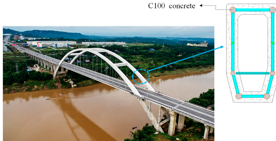
(a) View of Guansheng Qujiang Bridge.
