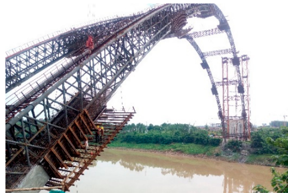
(c) Construction of reinforced concrete arch
