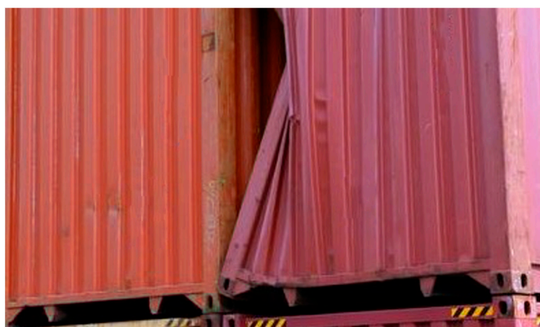
Figure 1. Example of a damaged marine container.
