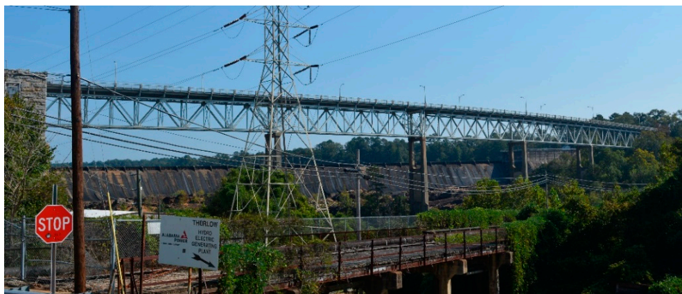
Figure 2. Fitzpatrick Bridge side view.
