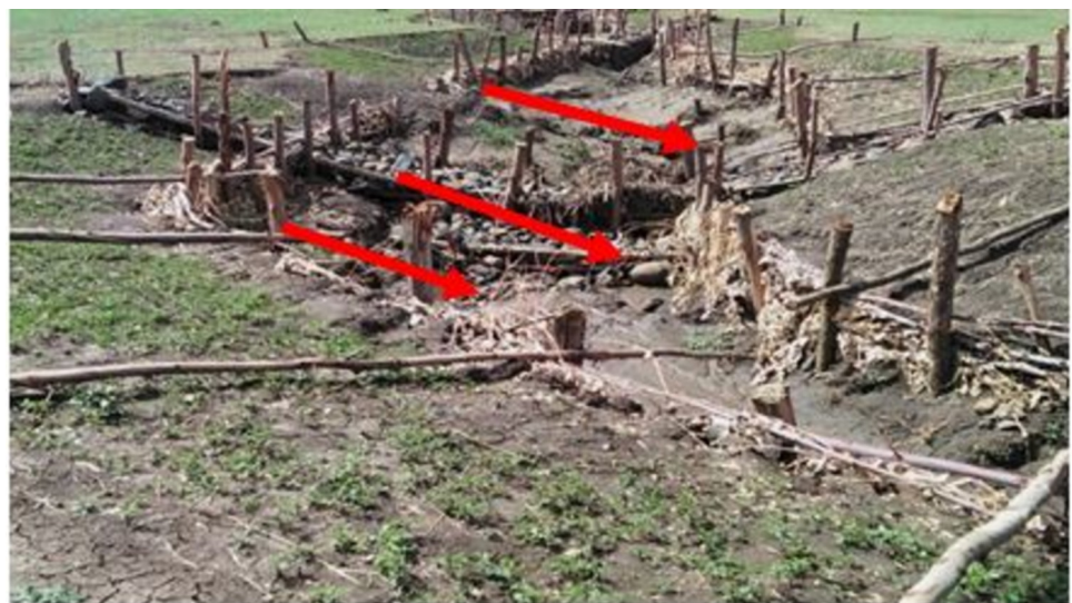
Fig 6. Brush wood check dam.
