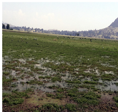
Figure 5. Wetland formed as a result of the dam construction.
