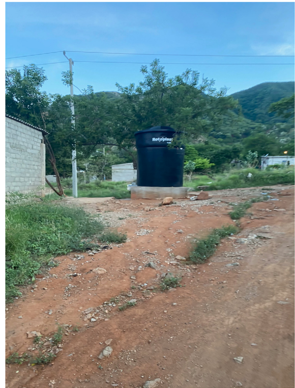
Figure 7. Water distribution tank.
