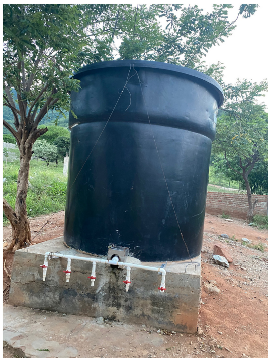
Figure 8. Front view of water distribution tank.
