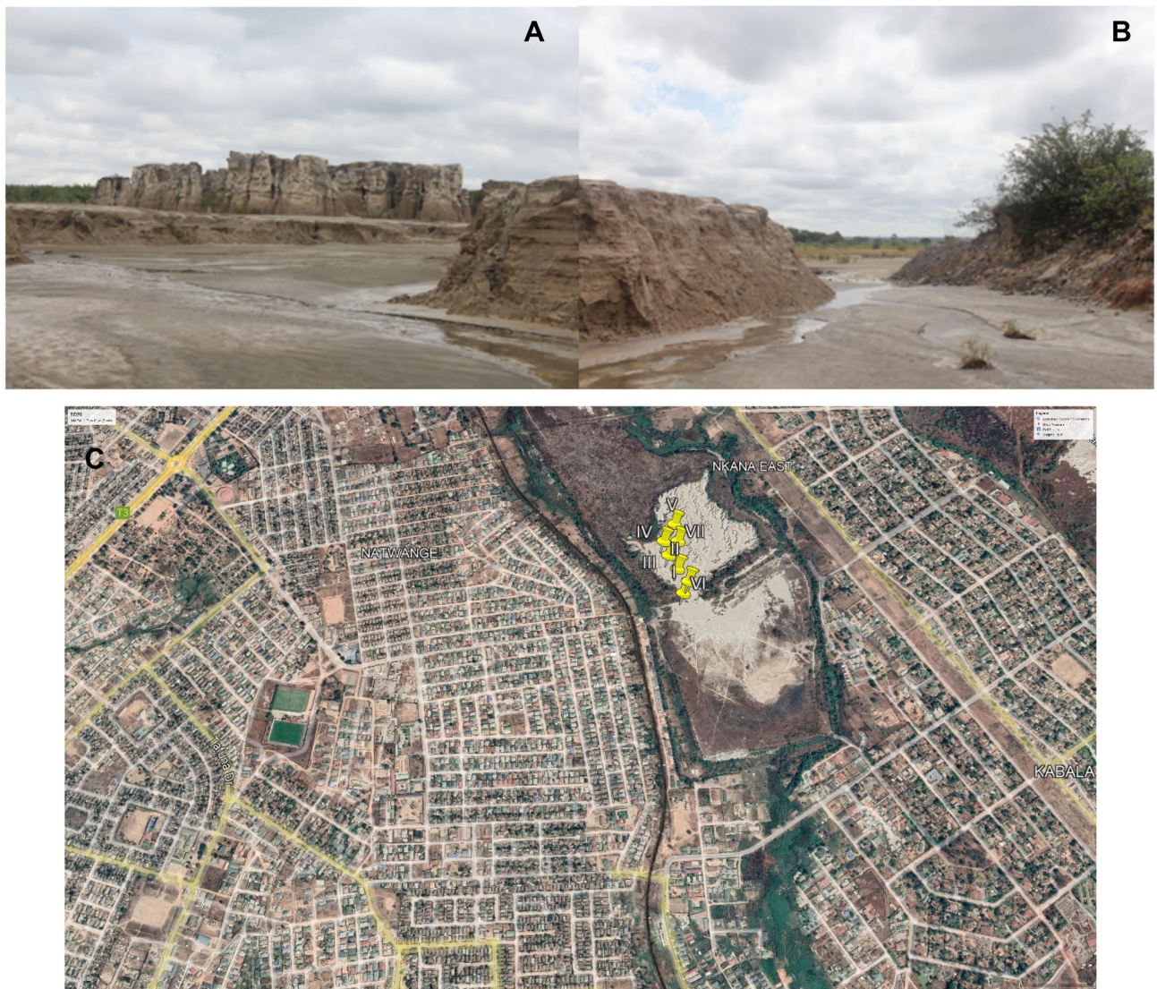
Figure 3. Uchi Tailing Dam (TD26). (A, B) Photographs showing compacted slurry on tailings, and gullies formed by water during the rainy seasons. The images: Leonce, June 2021. (C) An aerial photograph showing sampling points in yellow numbered I to VII at Uchi tailing dam location (TD26) and surrounding area, Google Earth Satellite Image system, January 2022.
